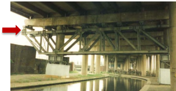
Temporary underpinning
